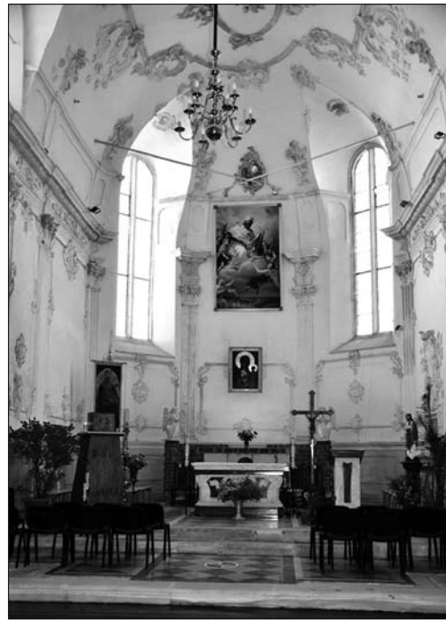
Fig. 2. Left-side asymmetry of the apse of the main altar (shift of pilasters with capitals to the left) in the Kamienets-Podilskyi church of St. Nicholas. Photo by the authors
